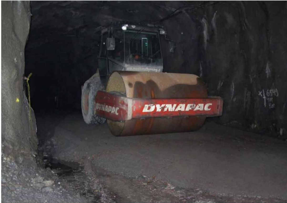
Ongoing preparation of road in production area.
