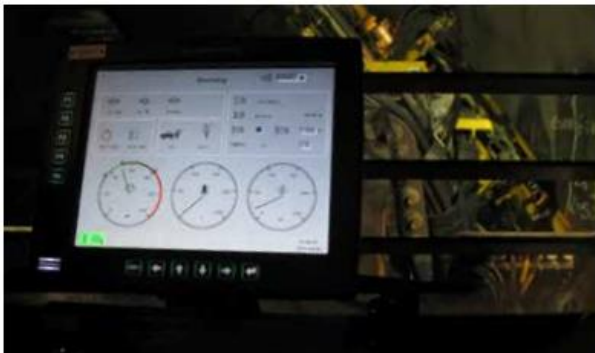
The Rig Control System (RCS) keeps deviation in drilling below 1.5%.
