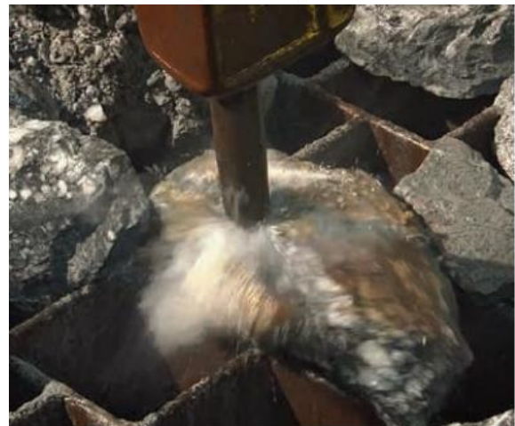
Breaking oversized rock is an essential task at crusher stations.
